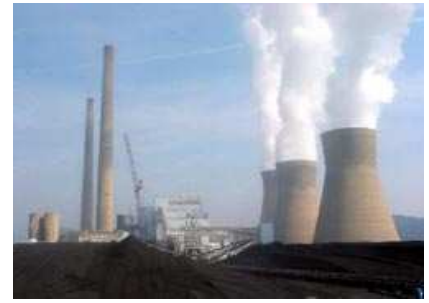
Coal Burning Power plant
